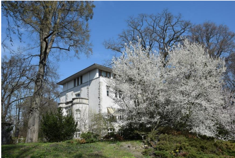
Main building of IGB at Lake Müggelsee. Photo: Nadja Neumann
